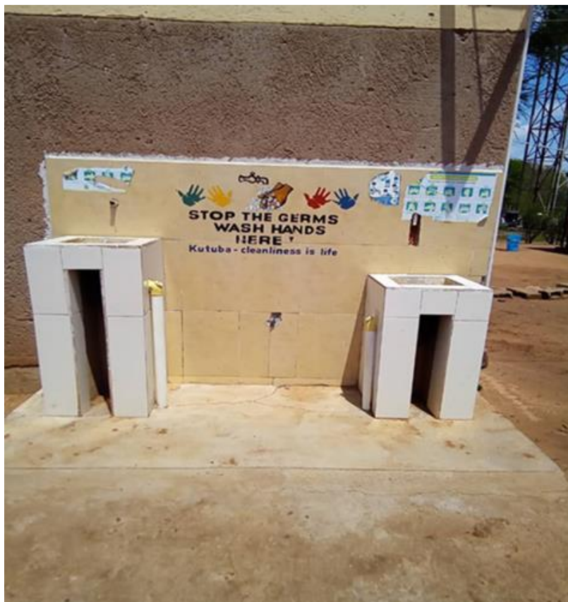
Figure 7: A handwashing facility at Mambova HCF without taps
